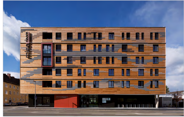
The OeAD residence minerroom in Leoben is the world's first large-scale timber passive house.
